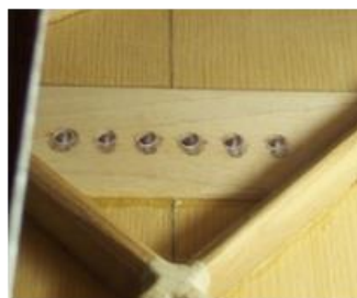
Example of a properly repaired bridgeplate on a 1953 Martin D-28. Pin hole damage to the original maple bridgeplate repaired in place with maple dust and hide glue.
